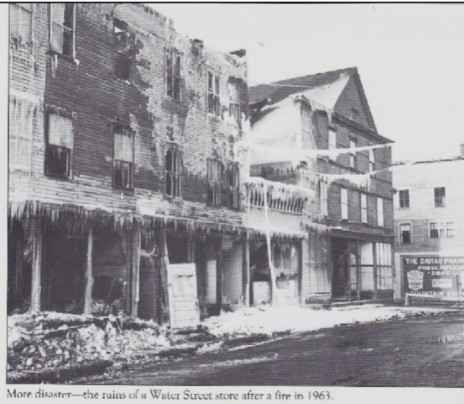
More disaster—the ruins of a Water Street store after a fire in 1963.
