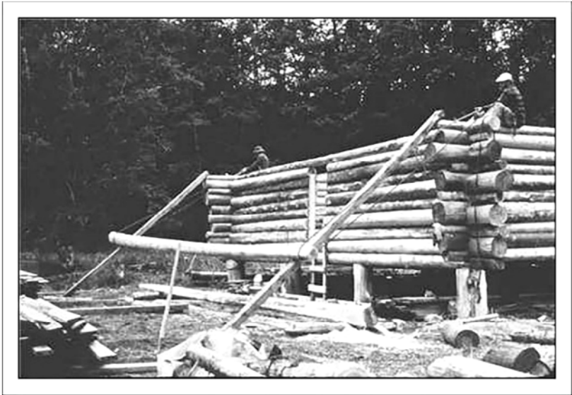
George (left) and Mike pull another log up a makeshift ramp to put into place.
