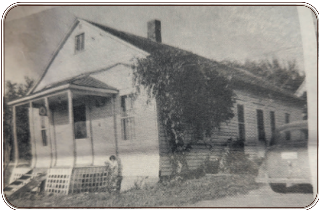
Gillett Grove's first telephone office building (aka Logan house). Ladies who served as Operators were Minnie Jorgensen, Mrs. Green, Arlene Logan, Darlene Stoermer and Thelma Lang. Photo credit: Gillett Grove Centennial Paper
